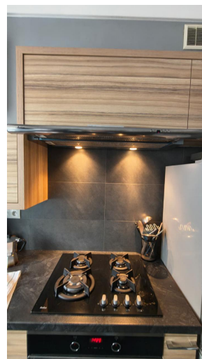
K12 Gas hob and under-cabinet extractor area.
